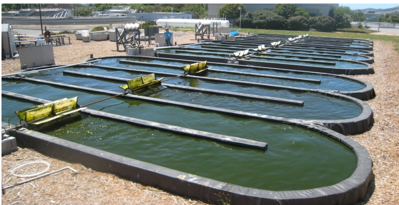
Figure 2. Suspended-growth ponds or raceways
