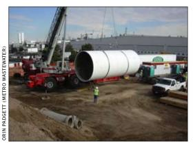
A Stanek Constructors Inc. (Denver) employee guides the first piece of fiberglass-reinforced pipe into place. Metro used 500 ft (152 m) of fiberglass-reinforced pipe in the design for the part of the conduit run that required a 50-year design life.
