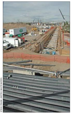
Last year, the Metro Wastewater Reclamation District (Denver) rehabilitated more than 1000 ft (305 m) of a reinforced concrete conduit with fiberglass-reinforced pipe. The project also required a 50-mgd (189,000-m<sup>3</sup>/d) bypass operation.
