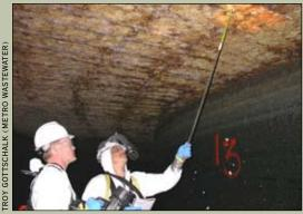
Orin Padgett, the Metro District's project manager, and Tim Volz of URS Corp. (Denver) inspect microbiologically-induced corrosion damage in the poured concrete box conduit that Metro rehabilitated.
