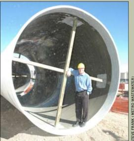
Norm Klapper, sales representative for Process Equipment Corp. (Boulder, Colo.) demonstrates the 11.2-ft (3.4-m) fiberglass-reinforced pipe used in the conduit rehabilitation. Each section weighs about 13,000 lb (5900 kg).
