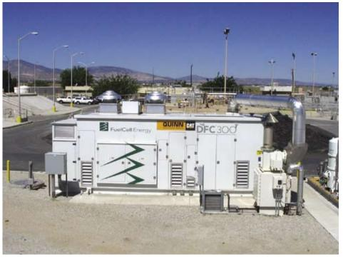
The 250-kW fuel cell at the Palmdale (Calif.) Water **Reclamation Plant** has an internal reformer, so digester gas can be injected directly into it.
