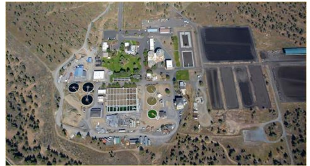
Bend Water Reclamation Facility on its 1,600-acre high-desert site
