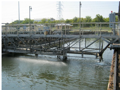
Village Creek WWTP, AL
