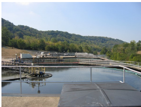
Figure 4— Octagonal Clarifier Configuration (Dry Creek WWTP, KY)
