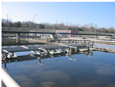
Clarksville WWTP, TN
