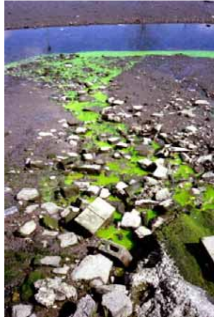
Dye tests to confirm improper sanitary sewage connection to storm drainage system SOURCE: Robert Pitt.
