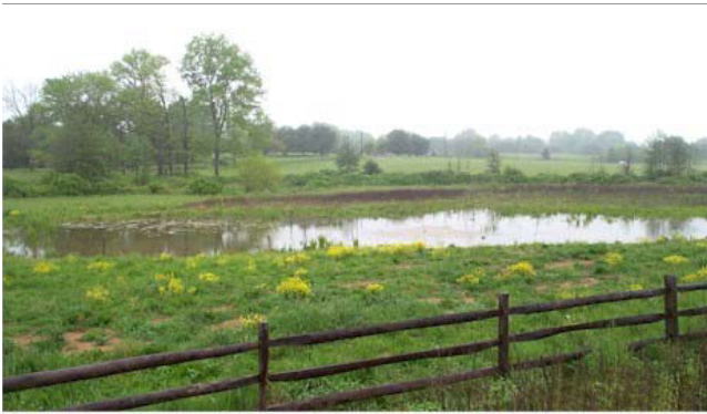
FIGURE 5-42 Wet pond. SOURCE: PaDEP (2006).
