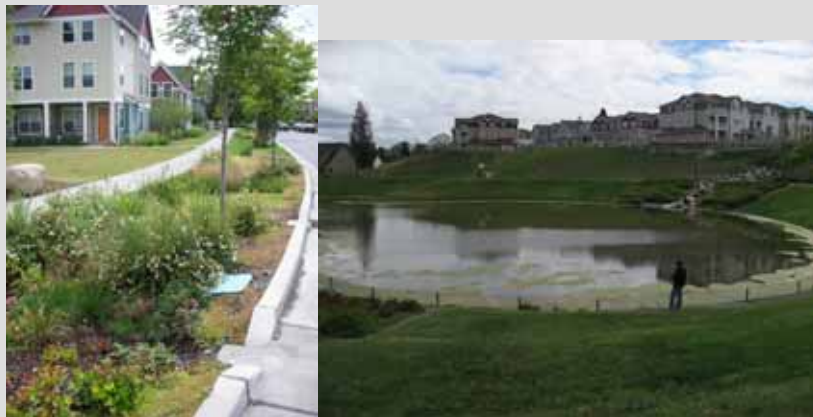
FIGURE 5-58 Natural drainage system methods have been applied to a 34-block, 1,600-unit mixed-income housing redevelopment project called High Point. Vegetated swales, porous concrete sidewalks, and frontyard rain gardens convey and treat stormwater on-site. On the right is the detention pond for the development.
