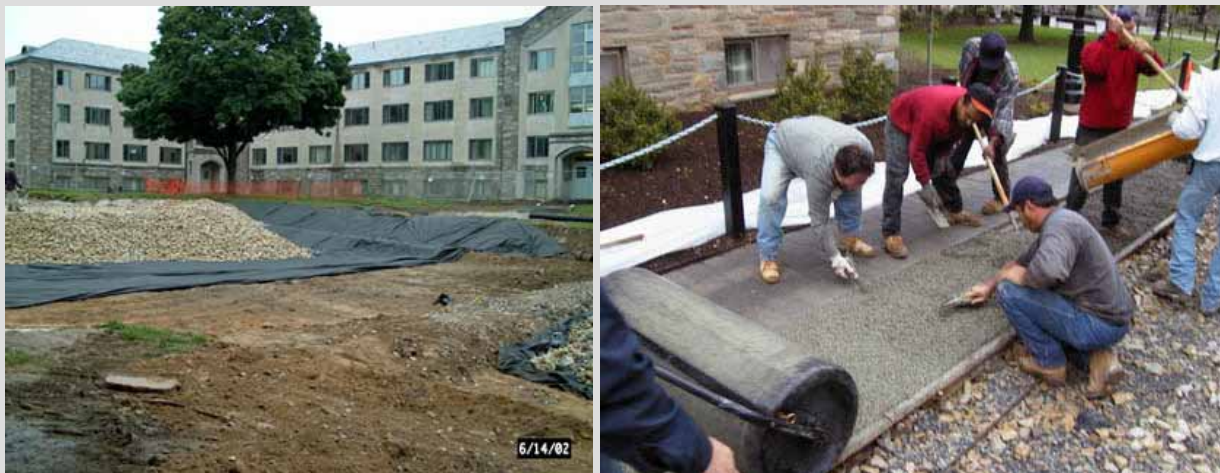
FIGURE 5-34 Infiltration bed under construction. Pervious concrete has functionality and workability similar to that of regular concrete. However, the pervious concrete mix lacks the sand and other fine particles found in regular concrete. This creates a significant amount of void space which allows water to flow relatively unobstructed through the concrete. This site was the first attempt at creating a pervious concrete SCM in the area, and there were construction and material problems. Since that time the industry has matured, and a second site on campus constructed in 2007 has not had any significant difficulties. SOURCE: Reprinted, with permission, from VUSP. Copyright by VUSP.
