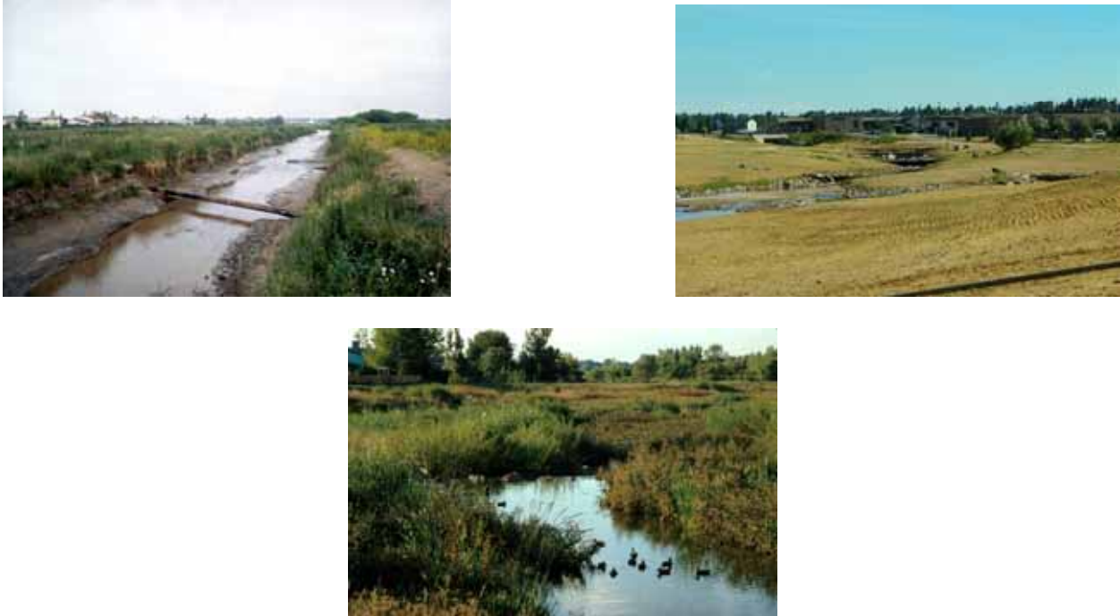
FIGURE 5-48 Three photographs illustrate stream rehabilitation in Denver. The top left picture is a creek that has eroded in its bed due to urbanization. The top right picture shows a portion of the stabilized creek immediately after construction. Check structures, which keep the creek from cutting its bed, are visible in the middle distance. The bottom image shows the creek just upstream of one of the check structures two years after stabilization. The thickets of willows established themselves naturally. The only revegetation performed was to seed the area for erosion control.
