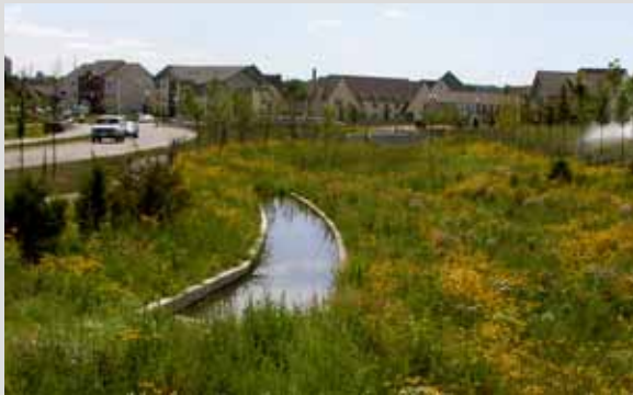
FIGURE 5-57 View of a sediment trap and porous landscape detention area in the central parkway spine of Heritage Park. The sediment trap in the center left of the photo was designed for ease of maintenance access by city crews with standard city maintenance equipment. Courtesy of SRF Consulting Group, Inc.
