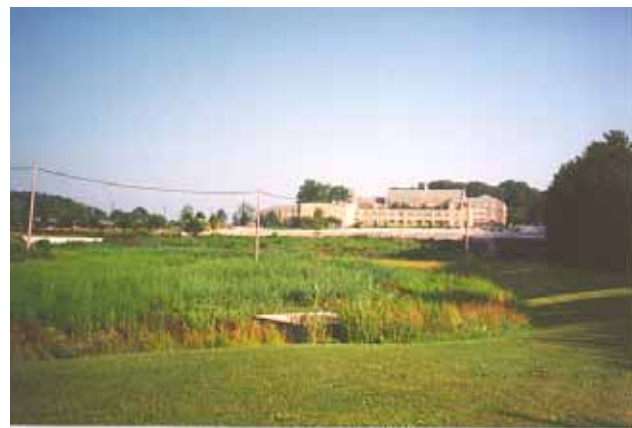
FIGURE 5-41 Retrofitted stormwater wetland. SOURCE: Reprinted, with permission, from VUSP. Copyright by VUSP.
