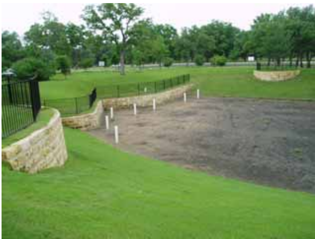
FIGURE 5-45 Austin sand filter. SOURCE: Robert Traver.
