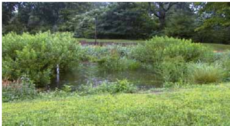
FIGURE 5-19 Retrofit bioinfiltration at Villanova University immediately following a storm event. SOURCE: Robert Traver.
