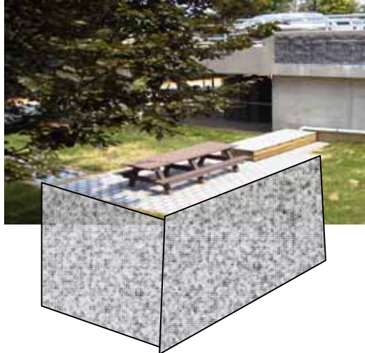
FIGURE 5-30 A retrofitted infiltration trench at Villanova University. SOURCE: Reprinted, with permission, from VUSP. Copyright by VUSP.
