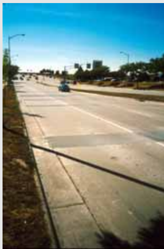
Wide arterial street with little roadside vegetation
