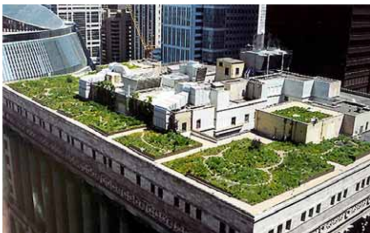
FIGURE 5-18 City Hall in the center of Chicago's downtown was retrofitted with a green roof to reduce the heat island effect, remove airborne pollutants, and attenuate stormwater flows as a demonstration of innovative stormwater management in an ultra-urban setting. SOURCE: Conservation Design Forum.
