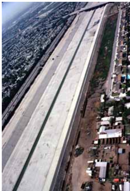
FIGURE 3-25 Example of a channelized urban stream for maximized flood conveyance and geomorphic stability (Los Angeles River, California). SOURCE: Reprinted, with permission, from Water Resources Research. Copyright by the American Geophysical Union.
