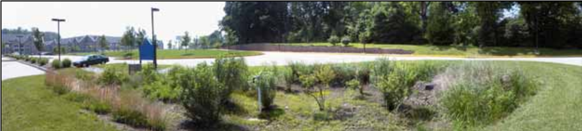
FIGURE 5-21 Villanova Bioinfiltration Traffic Island SCM. SOURCE : Reprinted, with permission, from VUSP. Copyright by Villanova Urban Stormwater Partnership.
