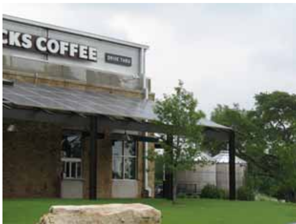
FIGURE 5-14 Rainwater harvesting tanks at a Starbucks in Austin, Texas. SOURCE: Laura Ehlers.
