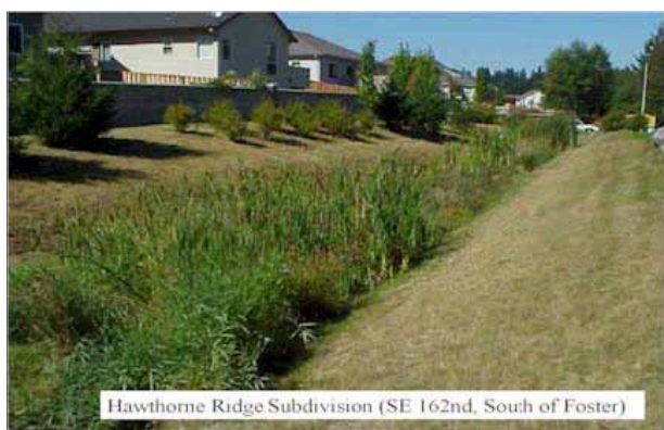
FIGURE 5-16 Vegetated swale. SOURCE: PaDEP (2006).
