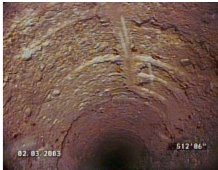
**Figure 4-2. Concrete pipe – Grade 4 (poor condition).**
