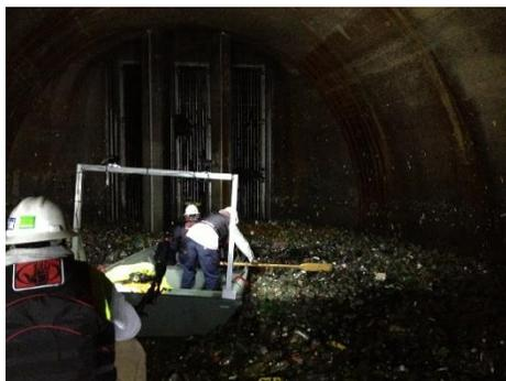
Figure 11 – Photo of operations staff removing floatables from a tunnel at Milwaukee MSD. (Photo provided by MMSD)
