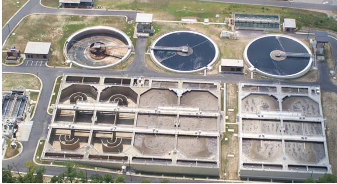
12 MGD Cary, NC BIO-DENIPHO Water Reclamation Facility
