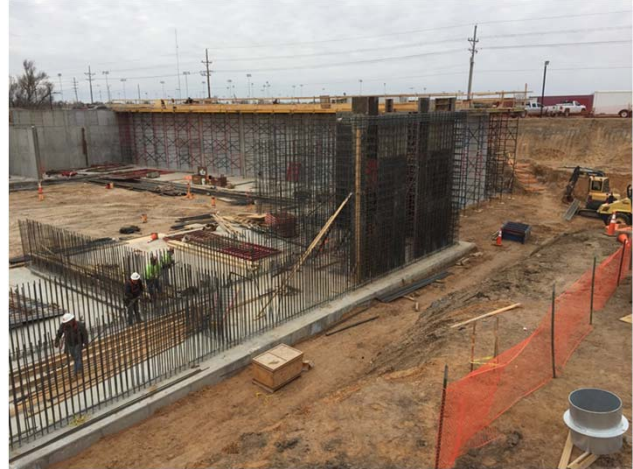
4.05 MGD BIO-DENIPHO Under Construction in Kansas
