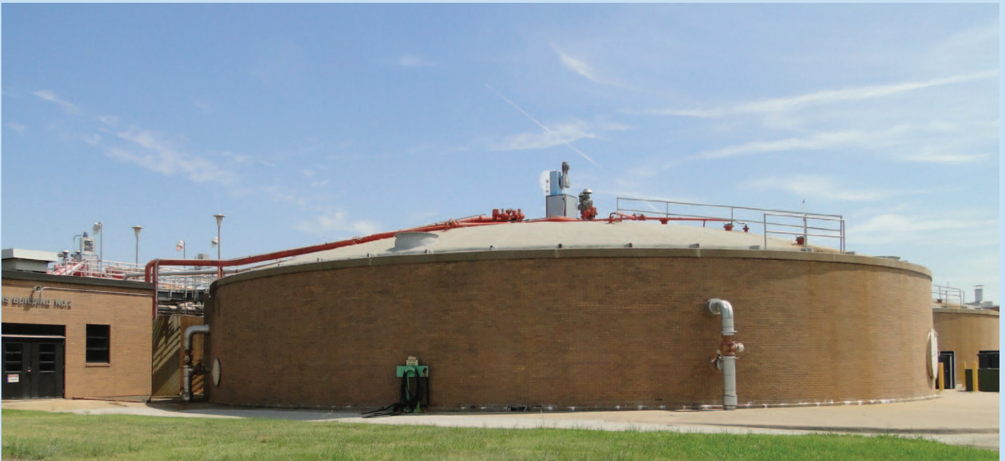
Top: Biogas, used to generate energy via the plant's turbines, is created in these anaerobic digesters fitted with linear motion mixers.
