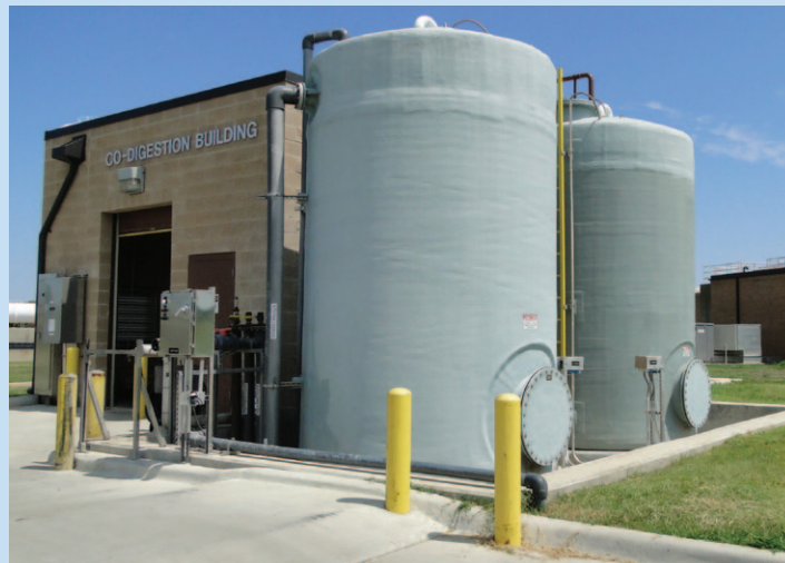
Top: Biogas, used to generate energy via the plant's turbines, is created in these anaerobic digesters fitted with linear motion mixers.
