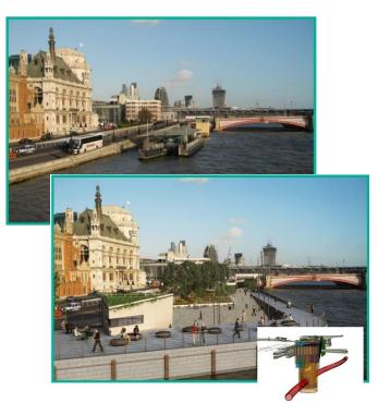
Figure 7 – Before and after for the Blackfriar drop shaft location along the Tideway Tunnel. Thames Water utilized green infrastructure to provide both a community walkway and tunnel access for operations staff. (Photo's provided by D. Crawford)
