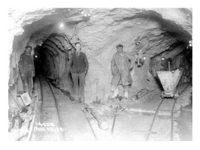
Figure 3 – Photo of workers constructing a connection between two sewer segments in an underground chamber of MWRDGC's Salt Creek Tunnel. (Photo provided by MWRDGC)
