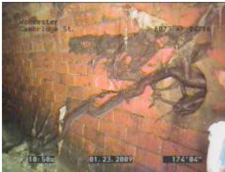
Figure 2-3. CCTV image of roots in lateral. Image courtesy of RedZone Robotics, Inc.
