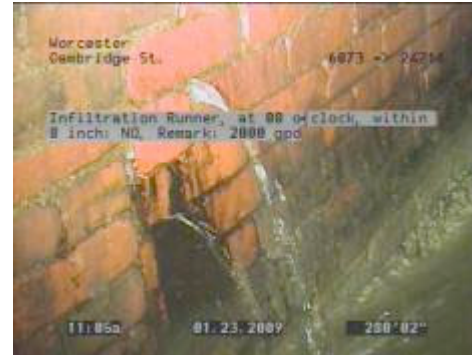
Figure 2-2. Example of infiltration. Image courtesy of RedZone Robotics, Inc.
