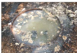
Blockage due to poor maintenance on Passive In-Ground Grease Traps
