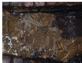
Grease from food preparation facilities caused blockages in a sewer line
