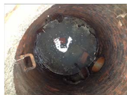
Grease in Manhole
