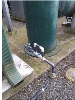
Duct drain
