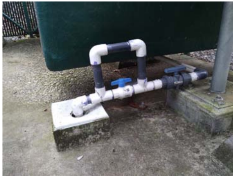
Mist eliminator drain
