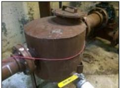
A close-up photograph of a cylindrical metal in-line strainer with a red band around it.
