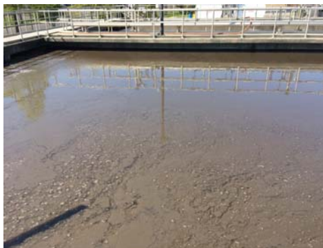
Anoxic Zone of Aeration Tank 8 Shown Above
