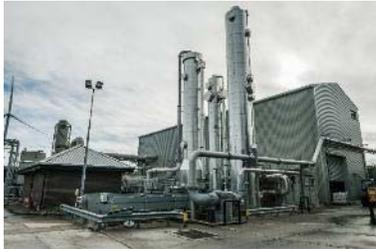
Biogas is purified to 98% methane through water-washing, upgraded with propane, and injected into the gas grid as direct substitute for natural gas
