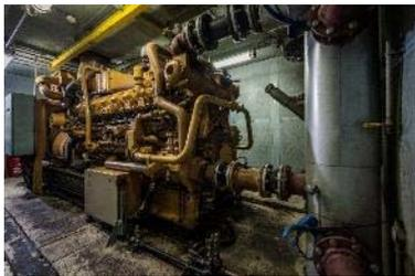
A portion of the site's biogas production is used in CHP engines to produce renewable electricity and heat for running the site
