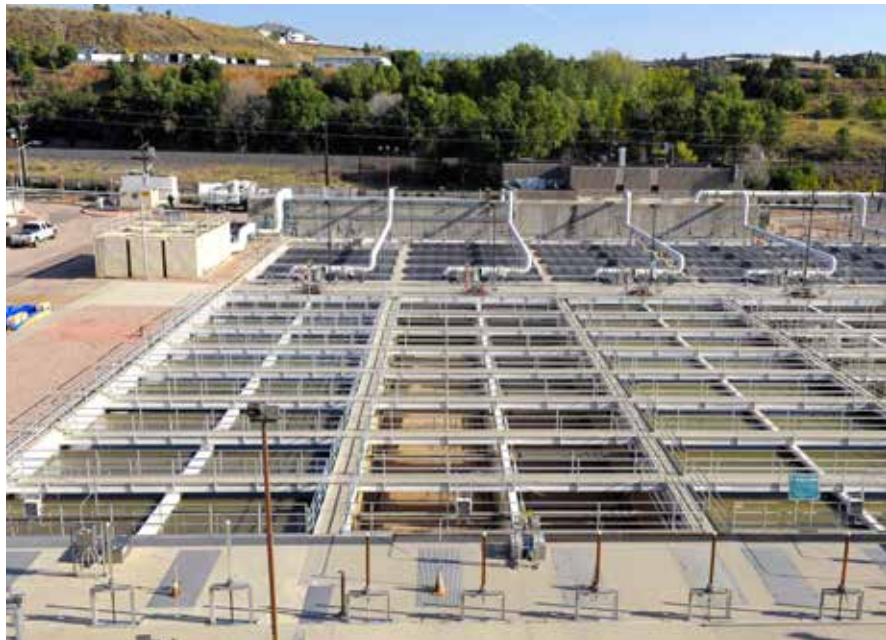
Primary sedimentation tanks remove suspended matter and floatables from the treatment process to prepare wastewater for additional treatment. Colorado Springs Utilities
