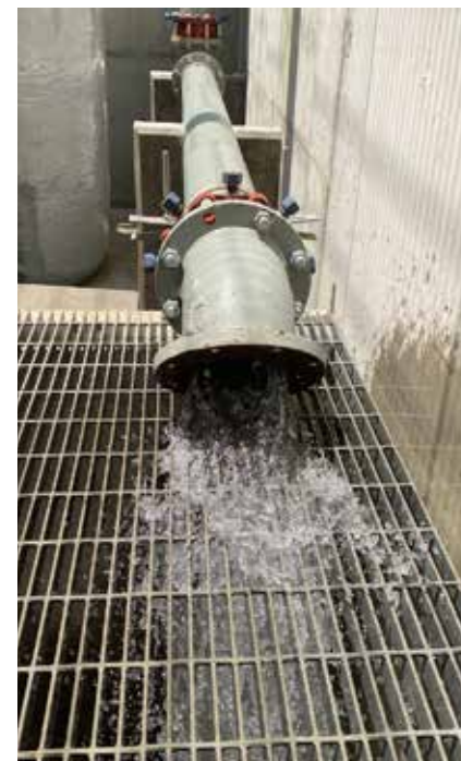
The stormwater harvesting system discharges where the treated water enters the cooling tower basin for use. University of Kentucky
