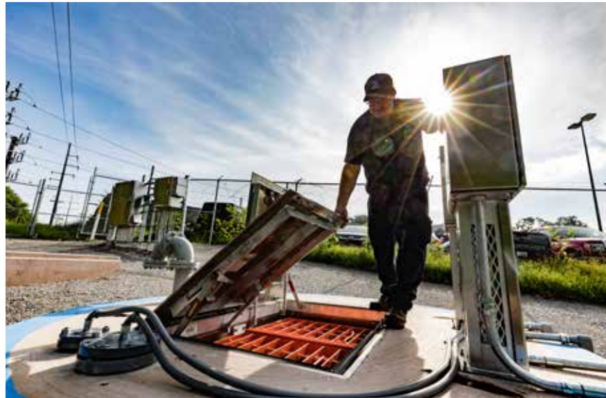
The stormwater harvesting wet well holds diverted stormwater for use in the University of Kentucky's Central Utility Plant, which is part of a chilled water loop used to air-condition campus buildings. Arden Barnes
